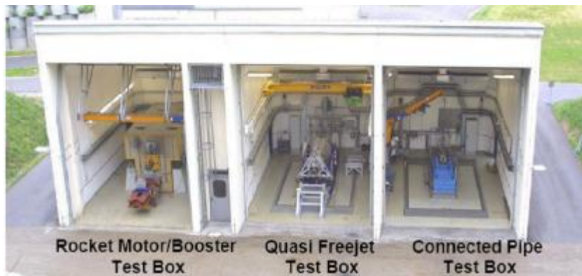
Figure 28: New test building for airbreathing motors at Aschau
